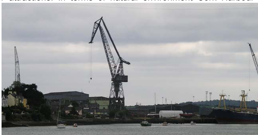
Cranes at Verolme Dockyard in Cork Harbour. Photo: Cathal O'Mahony.
